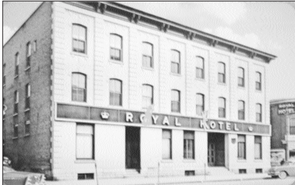
Above: The Royal as it appeared in the 1960s. The balcony extending from the second floor was removed earlier, and much of the brickwork and facade detail obscured by paint. This was much in keeping with the style of the time.
